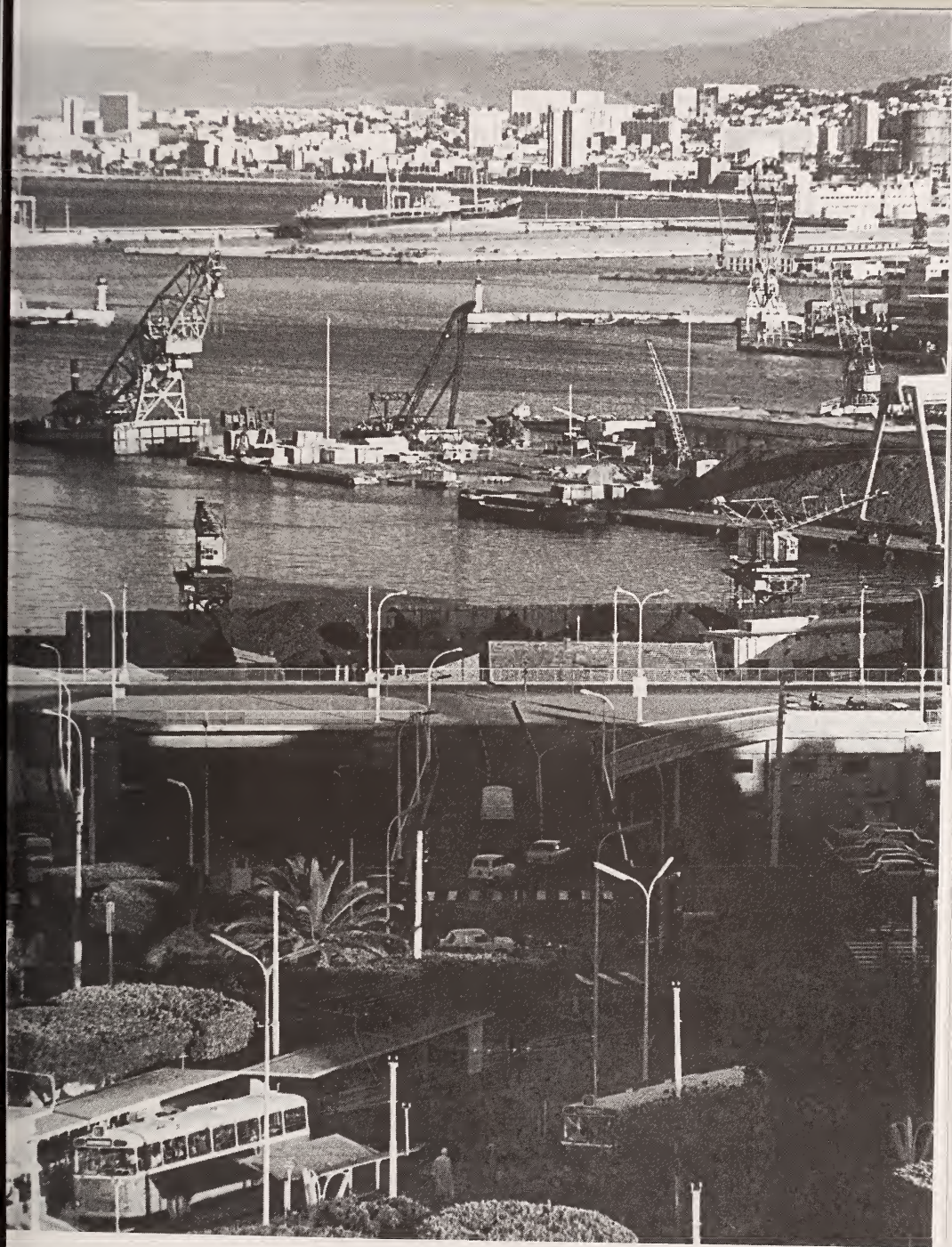
Port of Algiers, the country's principal maritime facility for general cargo and passengers Courtesy United Nations
